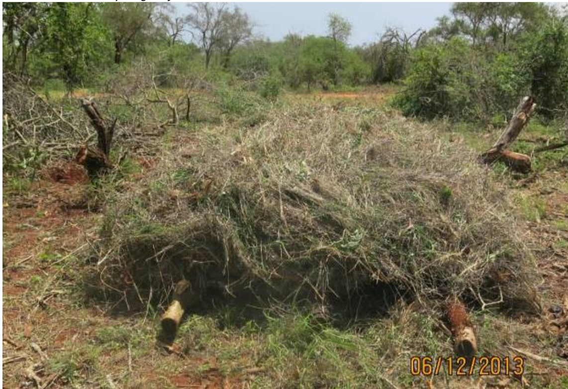
A charcoal kiln in early stages of construction
