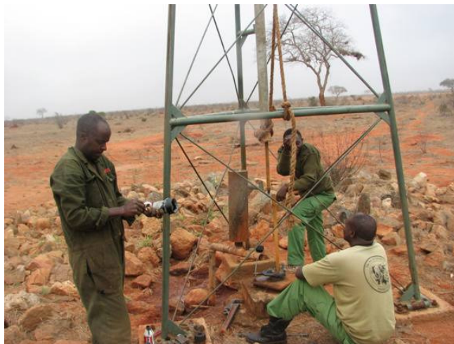
The Team assist with repair of the Dida harea windmill pump
