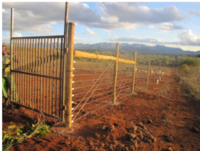
The fence line, phase 2
