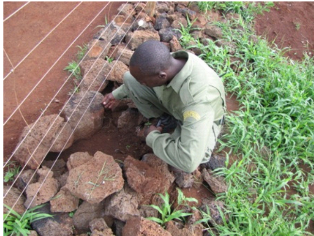
The Team checks for any signs of tampering on the new fence line
