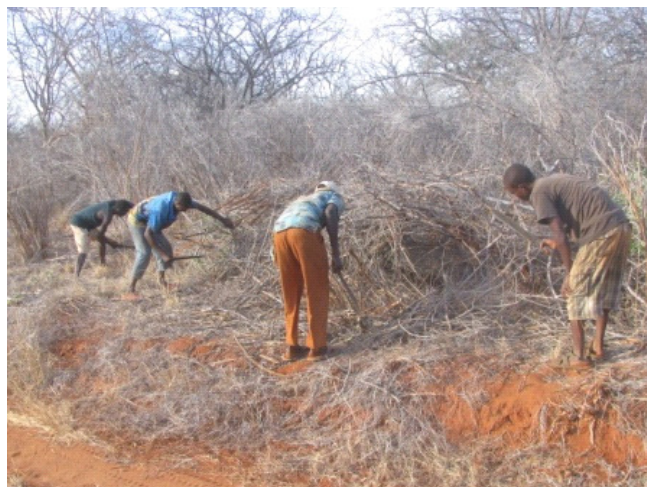
Casuals clearing the roads
